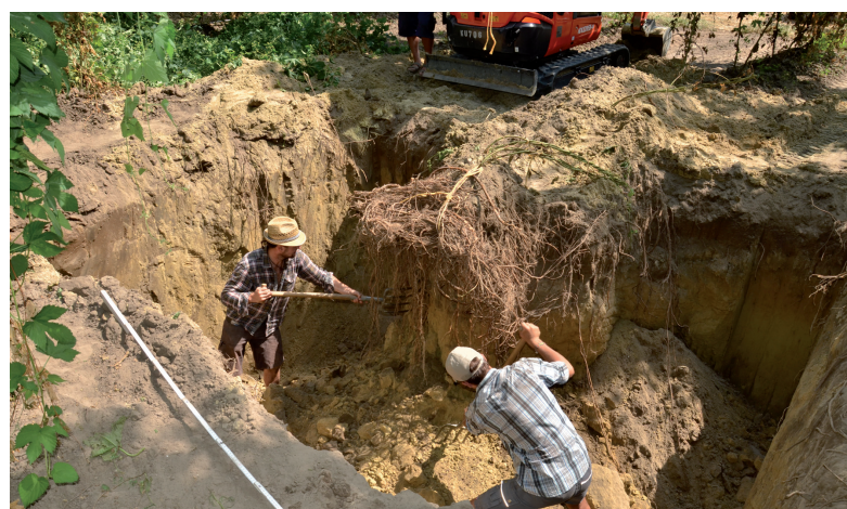
Fig. 1 Root excavation. The dimension of the trenched ditch was 3.8 x 3.2 m. Roots were prepared with digging forks
